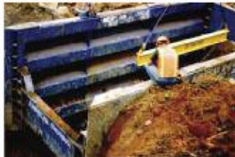
THE 10GLX1225 UNIT SHOWN HERE IS 12' HIGH X 25' LONG AND MADE OF HIGH ALLOY STEEL
