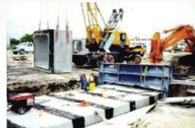
BOX CULVERT INSTALLATION WITH 18' HIGH X 18' WIDE CLEARANCES
