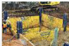
Remediation Slide Rail
