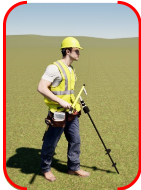
T-Handle and Socket is recommended to be used to install the temporary or temporal anchors
